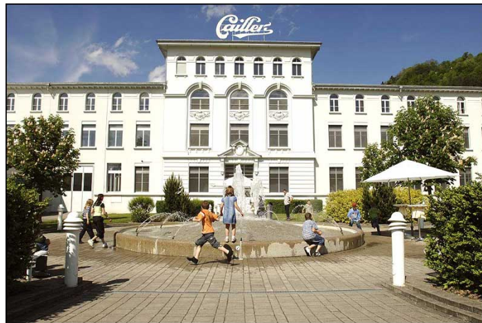
Picture 1: Maison Cailler, exterior view
